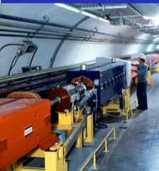
TUNNEL DEL SPS AL CERN
